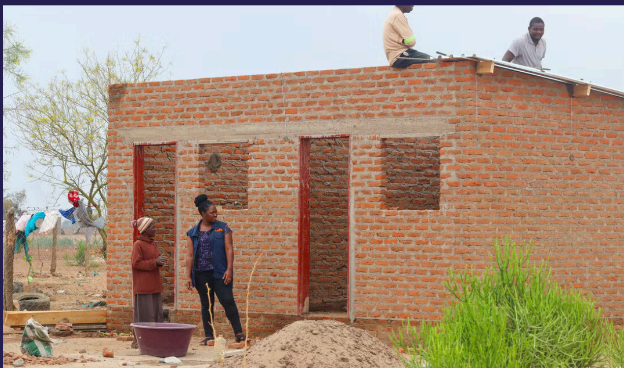
Two-room brick shelter construction in progress built by the community in Chipinge ©Pauline Hurungudo/CARE
