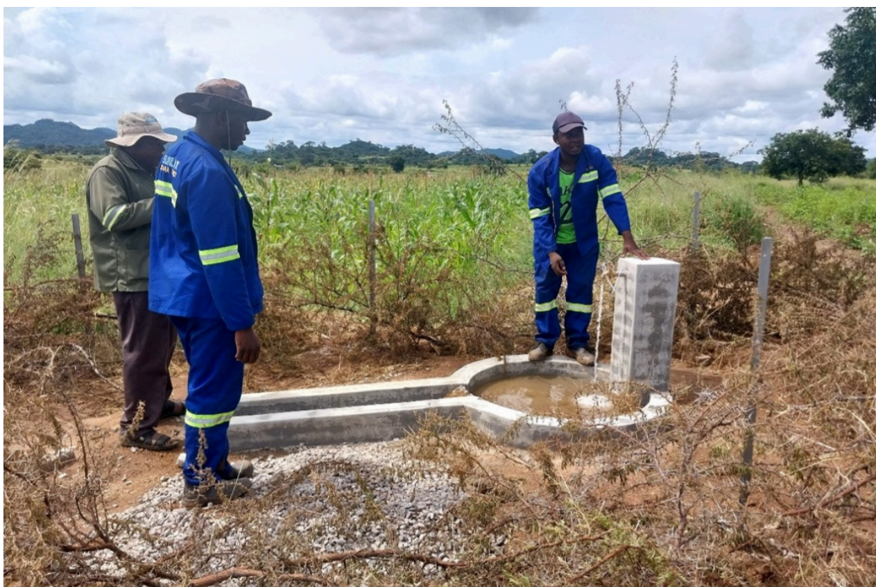
Builders examining the work just after completing a piped water point in Zaka Luxury Brand Crisis Modifier. ©Pauline Hurungudo/CARE Zimbabwe
